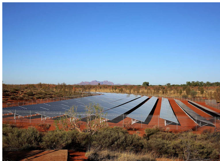
Photo. Yulara Solar project by Ark Energy
